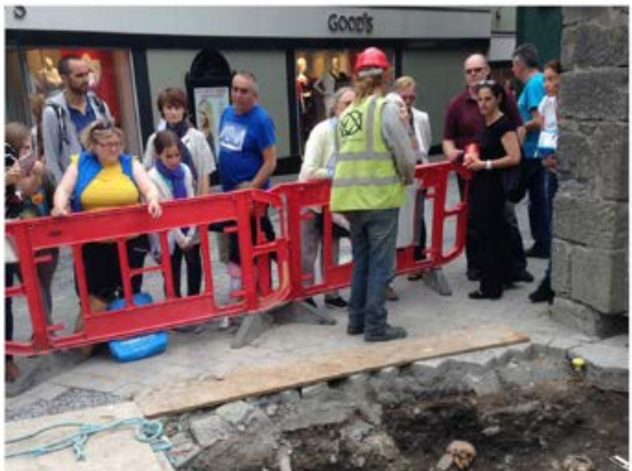
Excavation in Kilkenny City Centre - you can see skulls at the bottom right of the photograph.
